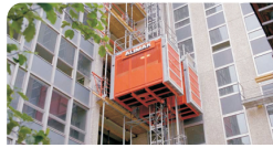
Construction Hoist
